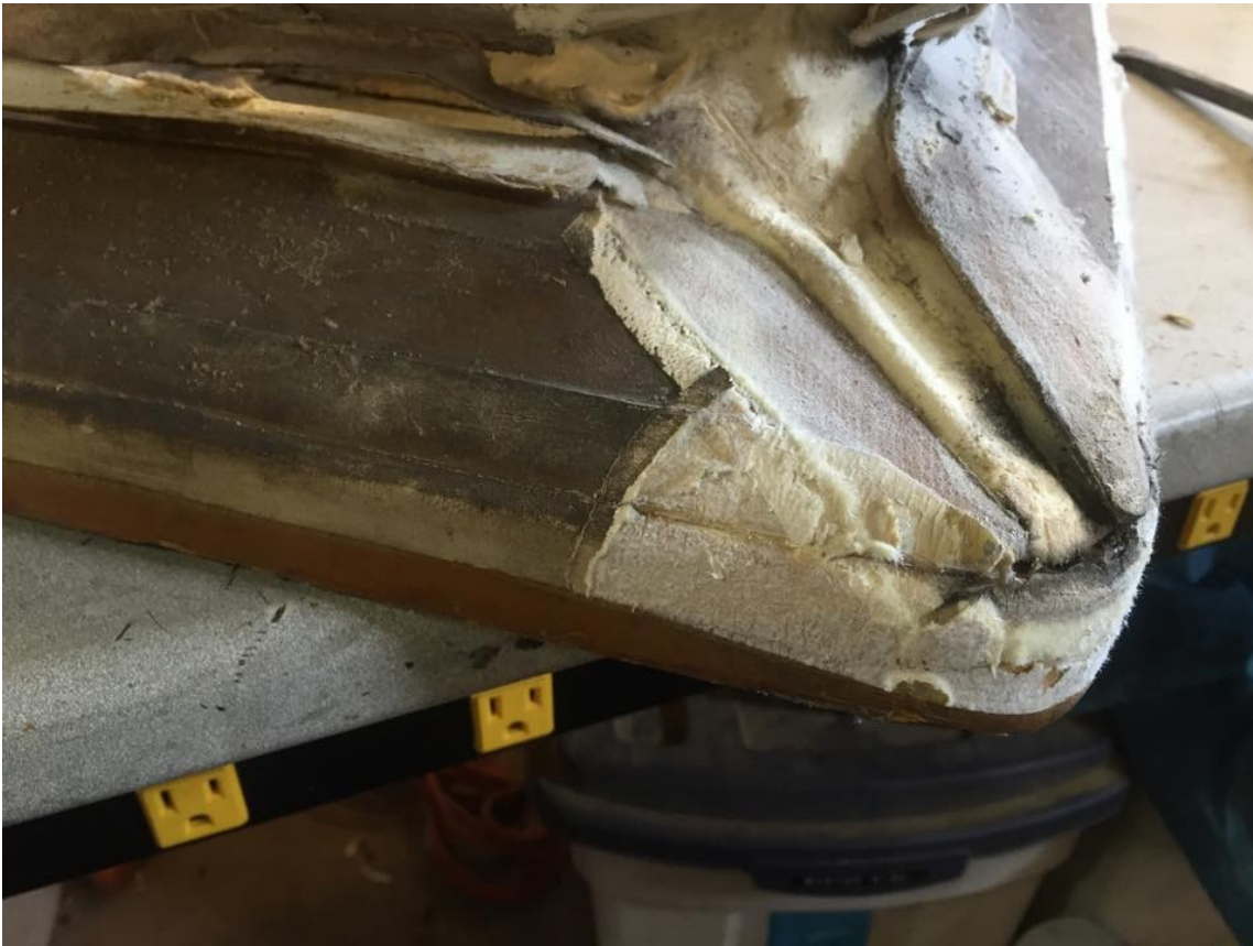
Left: Close-up of corner with outer gusset removed.
