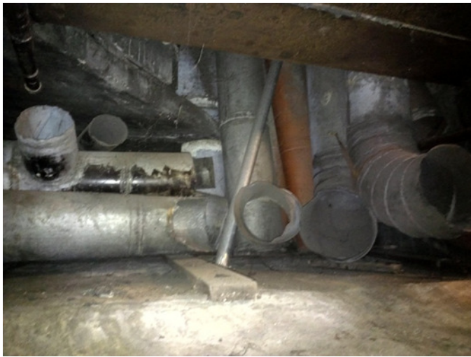
Above—wind lines stuffed into crawl spaces below the theater
